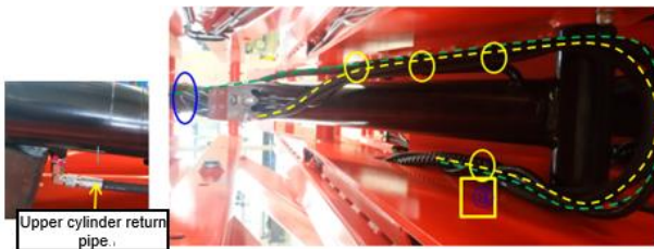
Fig. 4.90 Installation of third layer pipeline
